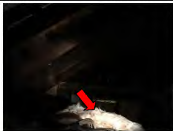
Photo 44. Roof space, Interior, Roof insulation, Insulation batts – Mineral wool SMF
