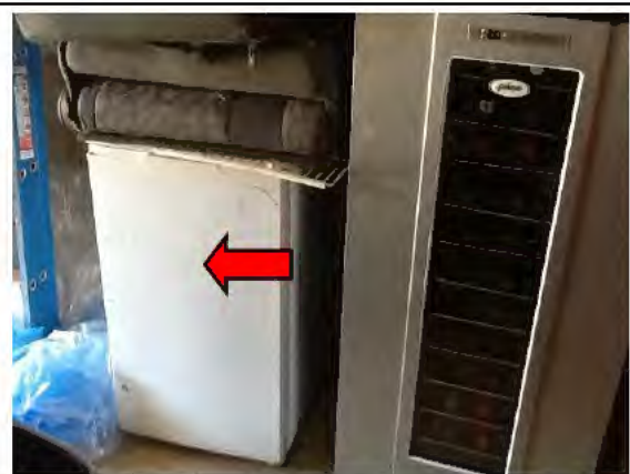
Photo 54. Level 0, Interior, Garage, Store Items, Refrigerator unit – Presumed positive for ODSs
