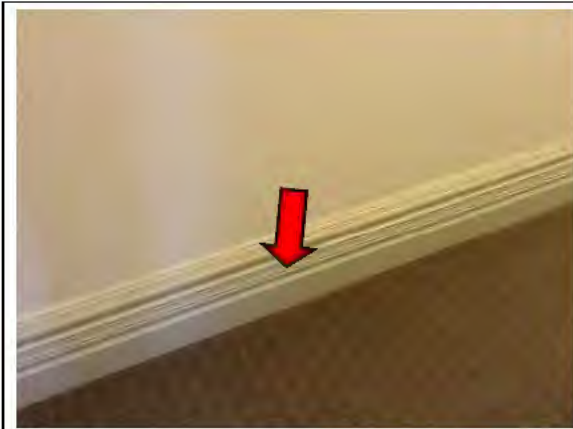
Photo 49. Levels 1 & 2, Interior, Skirting board/trim – Assumed lead-containing white lower coloured paint system
