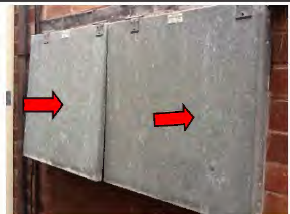
Photo 43. Level 1, Exterior, North wall, Switchboards – Presumed electrical backing boards
