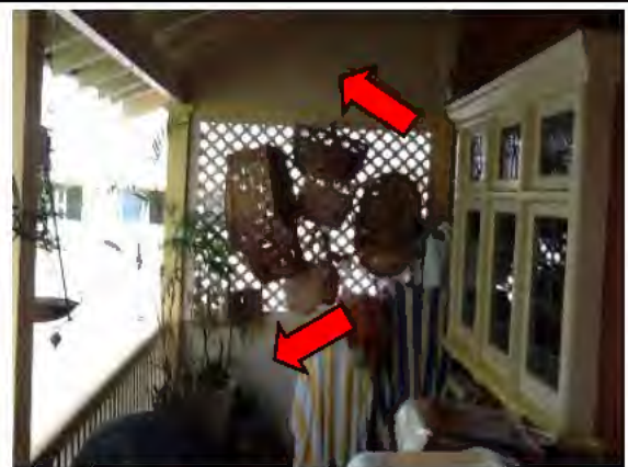
Photo 41. Level 2 (Flat no.1), Exterior, Northwest Balcony, North wall infill panels – Asbestos-containing fibre cement
