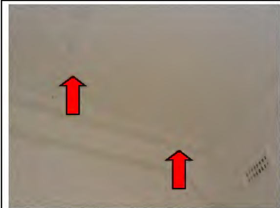
Photo 51. Levels 1 & 2, Interior, Ceiling, Coving and Décor trim – Assumed lead-containing white lower coloured paint system
