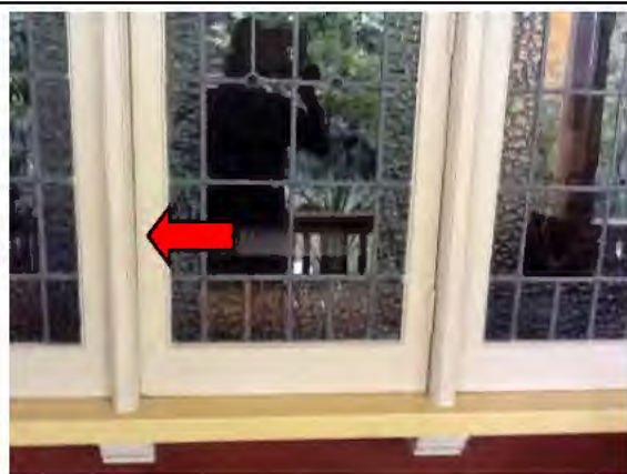
Photo 47. Levels 1 & 2, Exterior, Window frames – Lead-containing cream & yellow upper & white lower coloured paint systems
