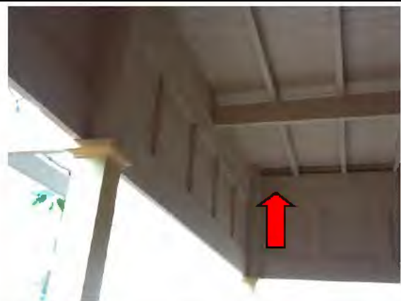
Photo 52. Level 1, Exterior, Timber work – Assumed lead-containing white lower coloured paint system
