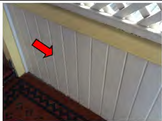
Photo 46. Levels 1 & 2, Exterior, Timber work – Lead-containing cream upper & white lower coloured paint systems
