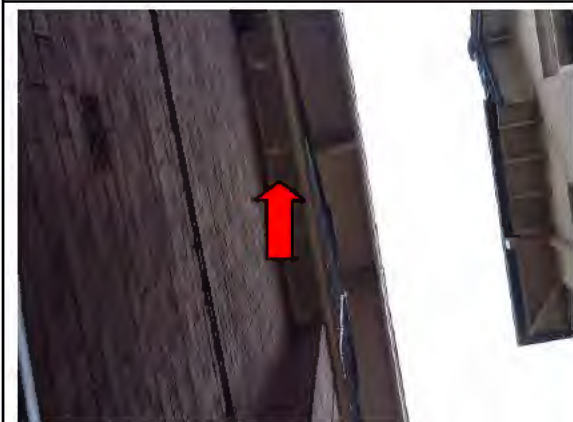
Photo 42. Level 2, Exterior, Roof, East, Eaves – Presumed compressed cement sheeting
