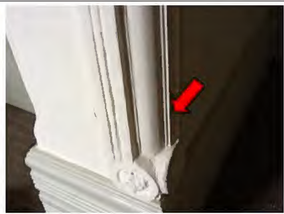
Photo 50. Levels 1 & 2, Interior, Walls, Décor trim – Lead-containing white lower coloured paint system
